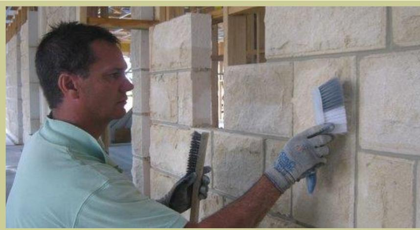
When mortar is evident on the stone wire brush off and then lightly dust again with a soft edge brush
