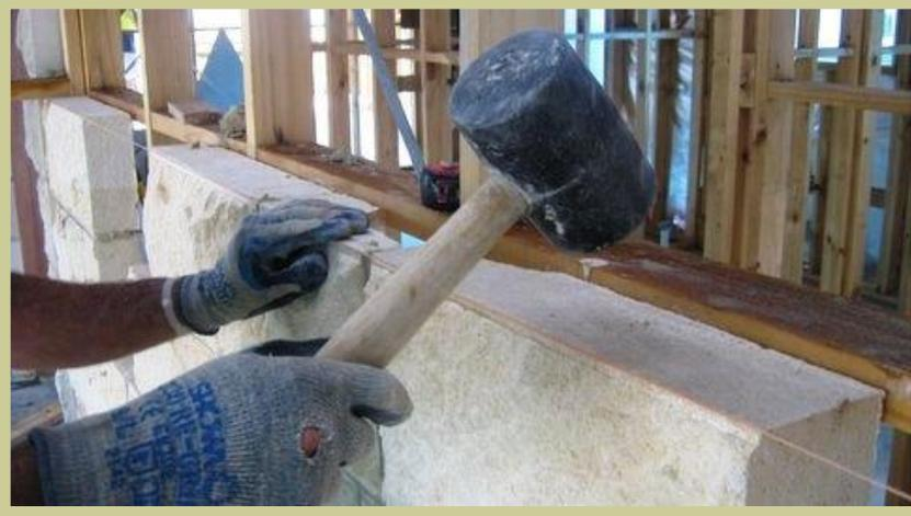
Avoid damaging the stone by using a rubber mallet to help keep stone in line with the stringline
