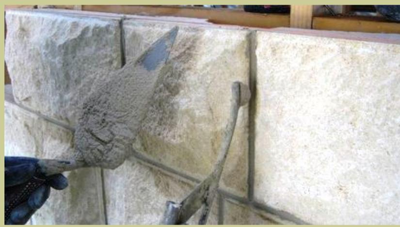
Point joints whilst mortar is still damp. Try to avoid mortar resting and drying on the stone
