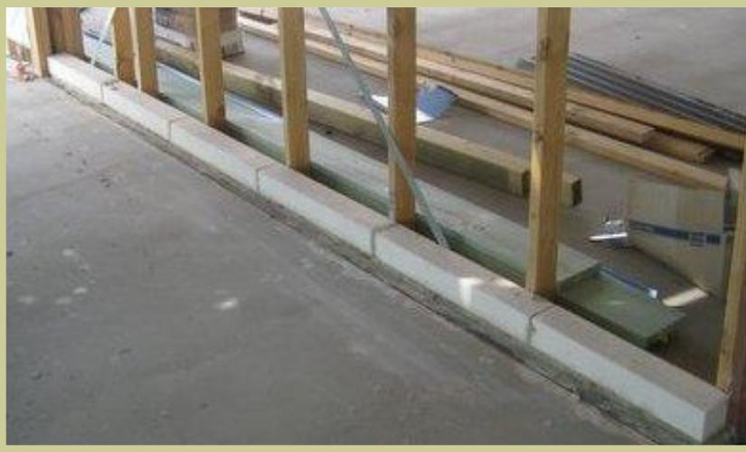
Lay the base stone completely square to ensure all other courses that follow are plumb. In this instance a plain face stone has been used as to offer a skirting effect on an internal wall
